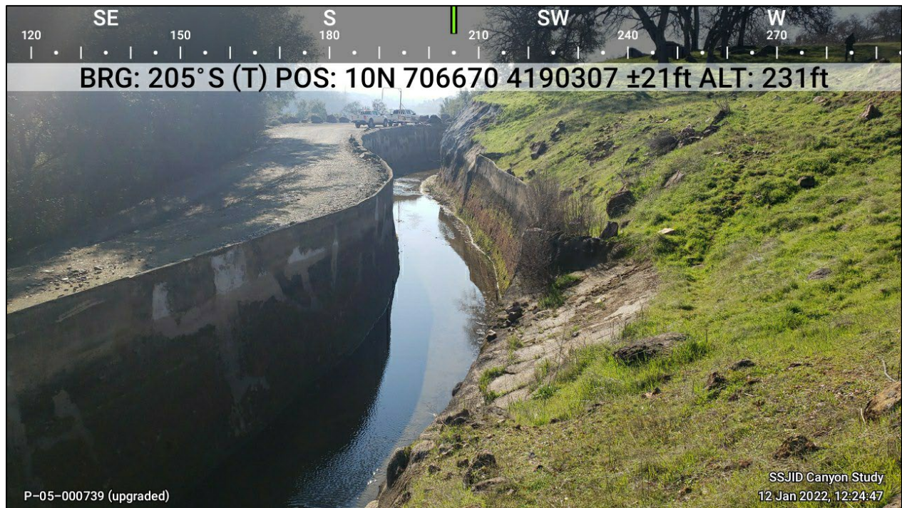
Figure 2. Recorded segment of P-5-000739/P-50-002109, looking south/southwest.
